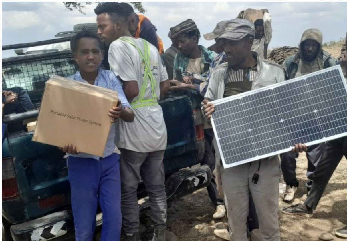
Picture 4 - Solar panel installation in Kembebet Woreda, Ethiopia
