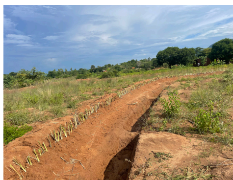
Snales and vetiver grass planted for flood and erosion protection
